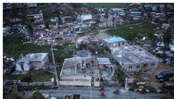
San Juan, PR after 5.8 earthquake
